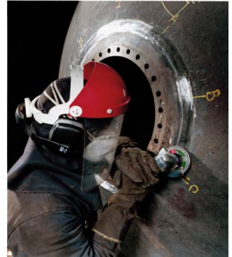
Zirc + in Action – finishing on stainless steel vessel
